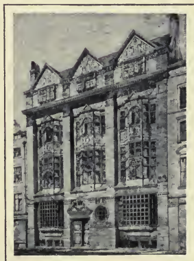
FIG. 225.—NEW ZEALAND CHAMBERS, LEADENHALL STREET. (NORMAN SHAW.)
