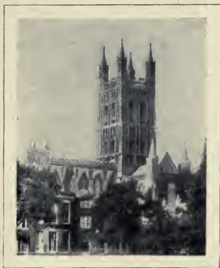
FIG. 137.—CENTRAL TOWER, GLOUCESTER CATHEDRAL.
