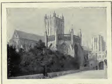
FIG. 94.—WELLS CATHEDRAL AND CHAPTER HOUSE, FROM THE NORTH EAST.
