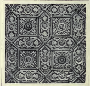
FIG. 144.—CEILING OF WOLSEY'S CLOSET, HAMPTON COURT.
