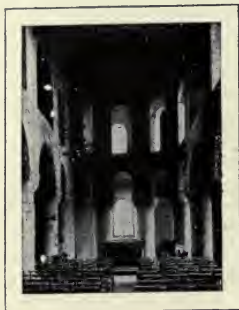
FIG. 39.—ST. JOHN'S CHAPEL, TOWER OF LONDON.
