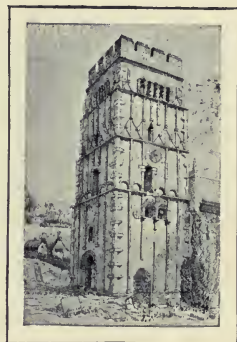
FIG. 24.—TOWER OF EARLS BARTON CHURCH, NORTHAMPTONSHIRE.
