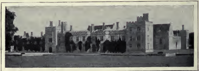
FIG. 105.—PENSURST PLACE, KENT.
