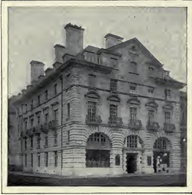
FIG. 241.—CHAMBERS IN ST. JAMES'S STREET. (NORMAN SHAW.)
