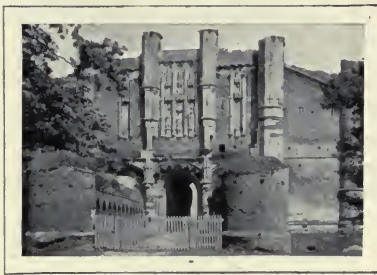
FIG. 132.—GATEHOUSE, THORNTON ABBEY.
